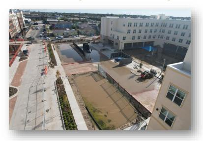
**Playground Issue:** Design issues relating to the existing soil on site not allowing water to properly drain through to underground drainage system.
